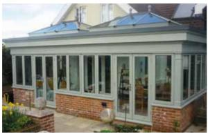
A frequently asked question "what is the difference between an Orangery and a Conservatory?" The main technical difference relates to how the roof of each is constructed. A very simple differentiation is that a conservatory has the majority of its roof glazed, whereas an orangery tends to have a solid perimeter roof with roof lanterns to allow light in.
